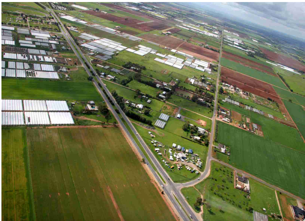
Intersection of Port Wakefield Road and Taylors Road looking north-east
